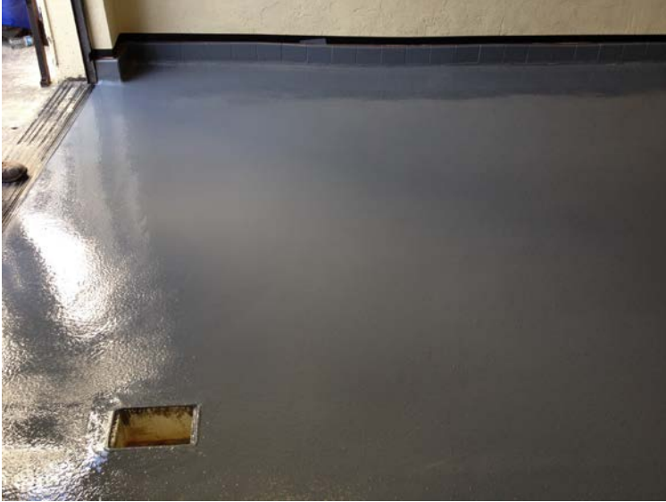
Seamless transition to floor sink
