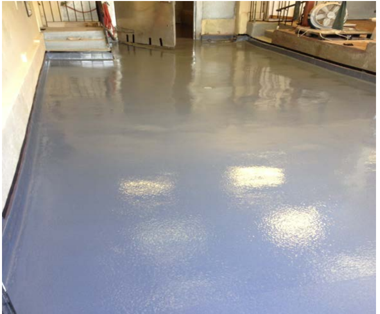
Chemical & abrasion resistant 100% solids epoxy in dark grey
