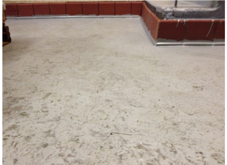
Scratch coat plus cementitious urethane slurry rated for forklift traffic
