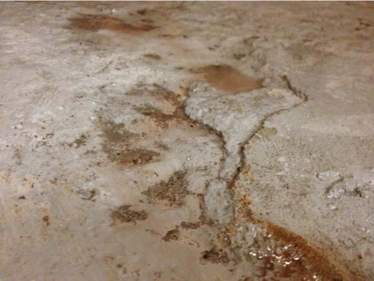
Degreased; diamond grinding and shot blasting substrate in progress
