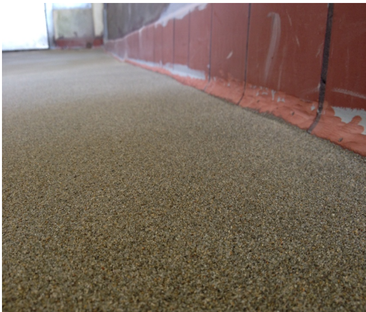
Cove tiles have been ground down for seamless transition
