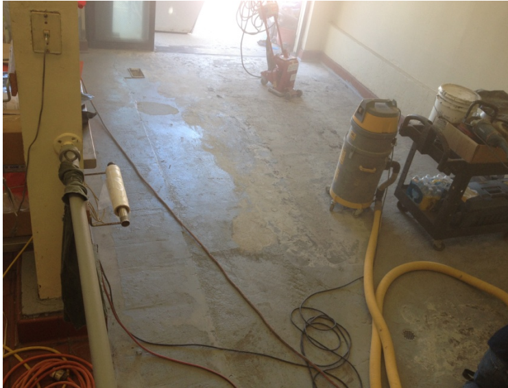
Cove tiles have been ground down for seamless transition
