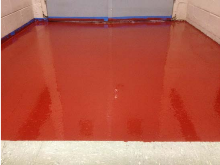
1/4" trowel down urethane slurry with epoxy seal coat
