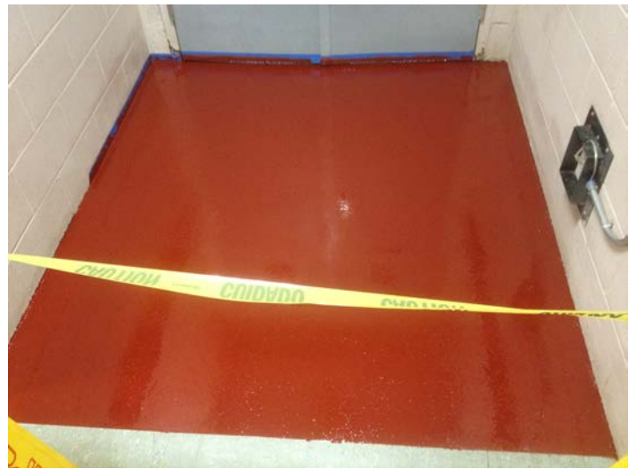
Removed all overlays, glues & cleaned with microbial
