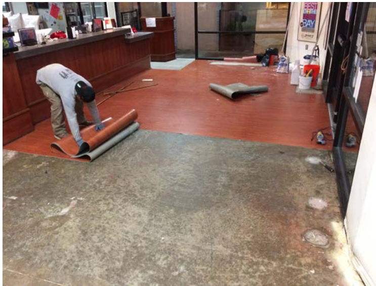
All clean, mechanically prepared & scrubbed clean
