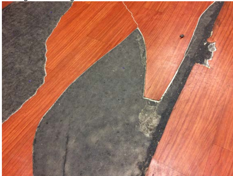
Next diamond grind whole area & edges to prepare for seal coat
