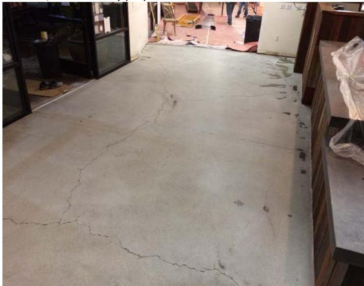
All clean, mechanically prepared & scrubbed clean
