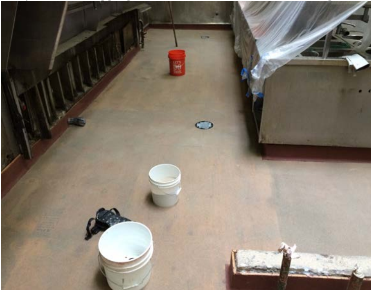
Body coat with aggregate to ensure mechanical bonding of subsequent layer. Trowel install 1/4" cementitious urethane mixture
