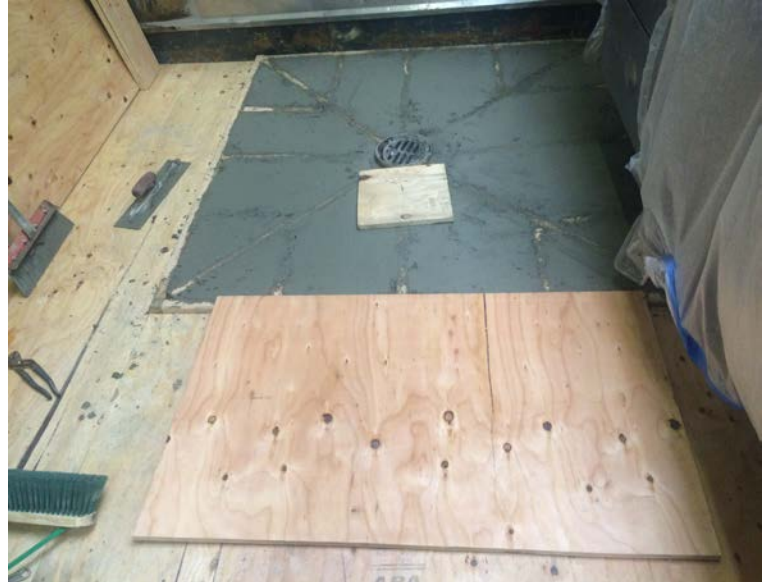
Subfloor started with waterproofing cement around drains
