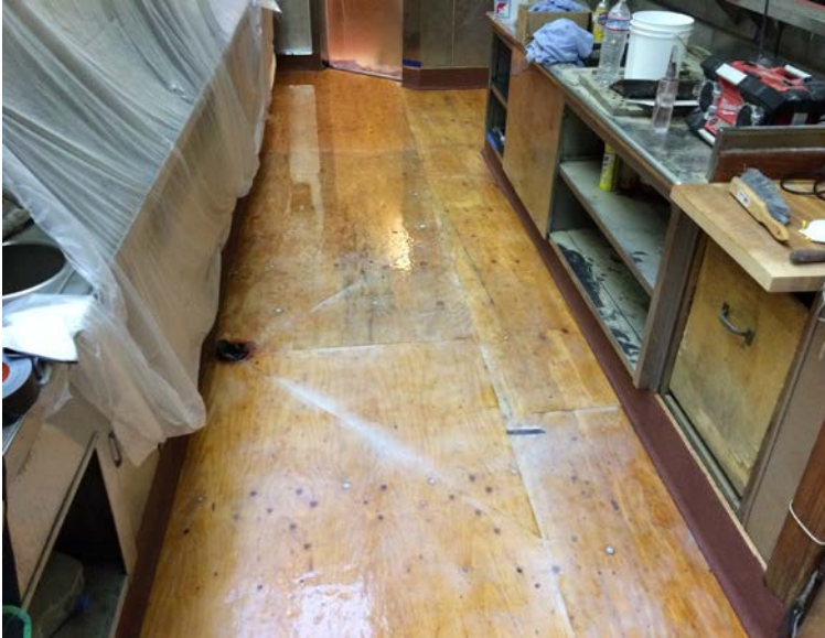
Body coat with aggregate to ensure mechanical bonding of subsequent layer. Trowel install 1/4" cementitious urethane mixture
