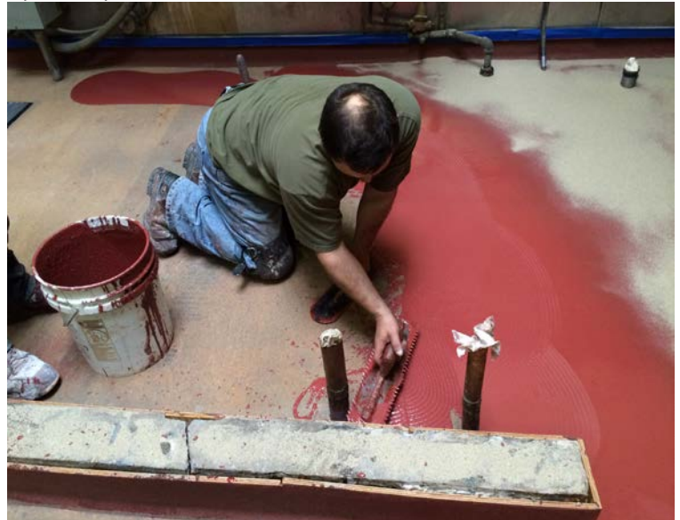
Body coat with aggregate to ensure mechanical bonding of subsequent layer. Trowel install 1/4" cementitious urethane mixture
