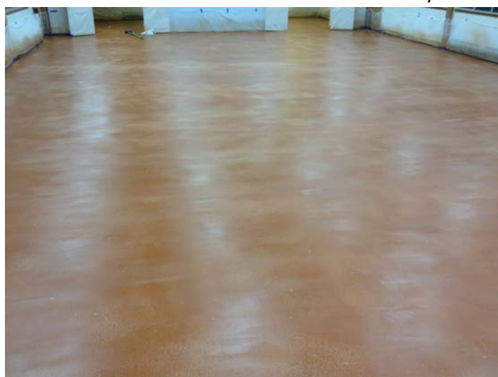
Base coat of Terra Cotta after cementitious overlay
