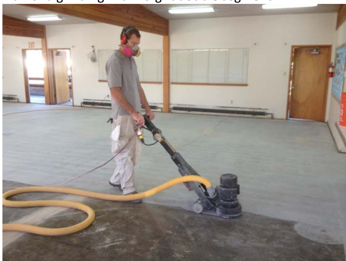
Diamond grinding with 16-grit double segment
