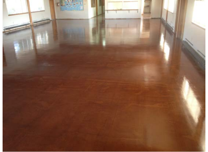
Project finished with sealer
