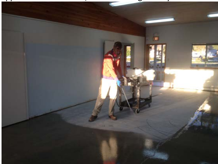
Application of densifier/moisture mitigation system
