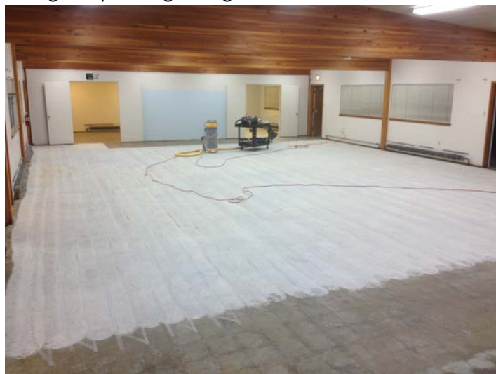
During first pass of grinding
