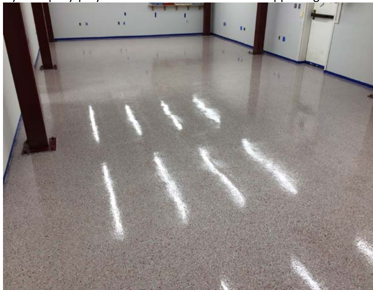
Hybrid epoxy-polyurethane makes for durable & appealing finish
