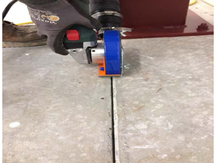
Control joints, cracks, bolt holes & imperfections all being repaired
