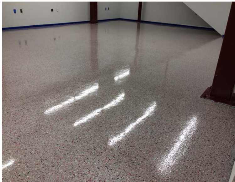
Hybrid epoxy-polyurethane makes for durable & appealing finish
