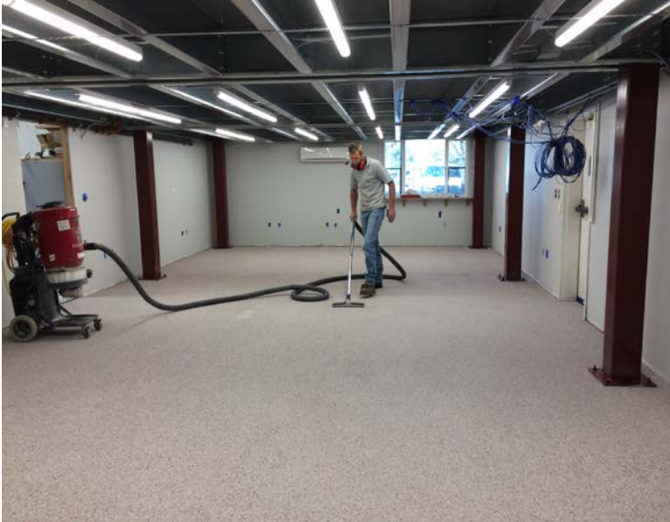
Scraped, then vacuum excess decorative vinyl flakes prior to topcoat
