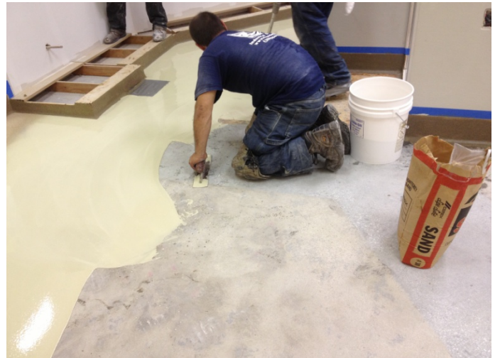
Back-roll to prevent outgassing
