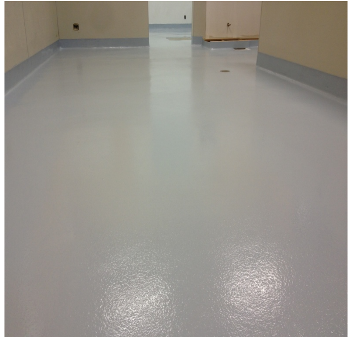
Kitchen and food preparation areas completed
