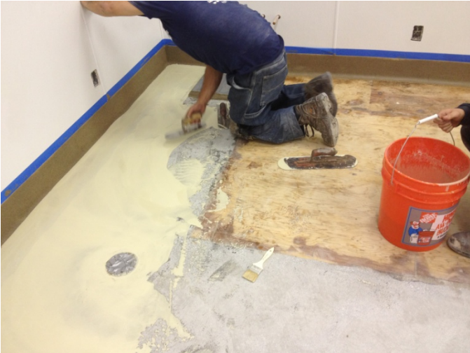
Trowel apply 3/16" cementitious urethane
