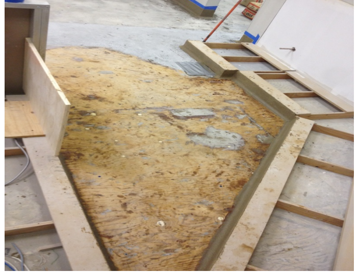
Over plywood & concrete substrate
