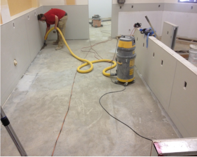
Diamond grind etches & corners
