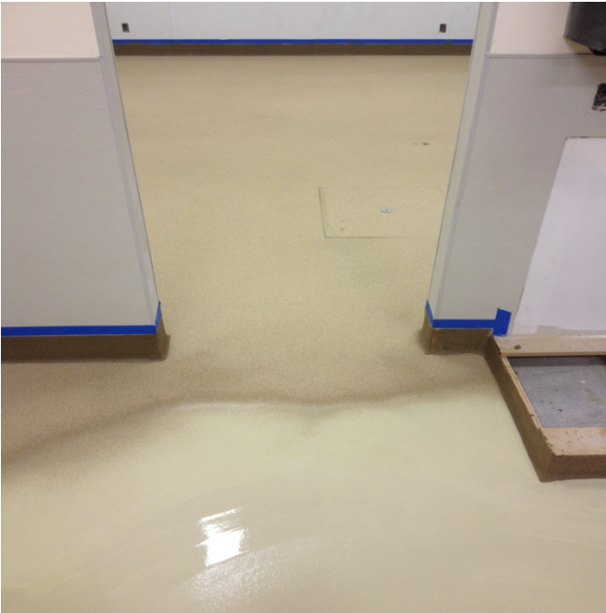
Broadcast sand to rejection for non-skid & more impact resistance
