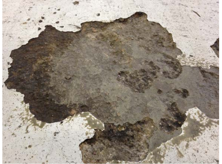
Chemical & abrasion resistant topcoat of moisture tolerant floor
