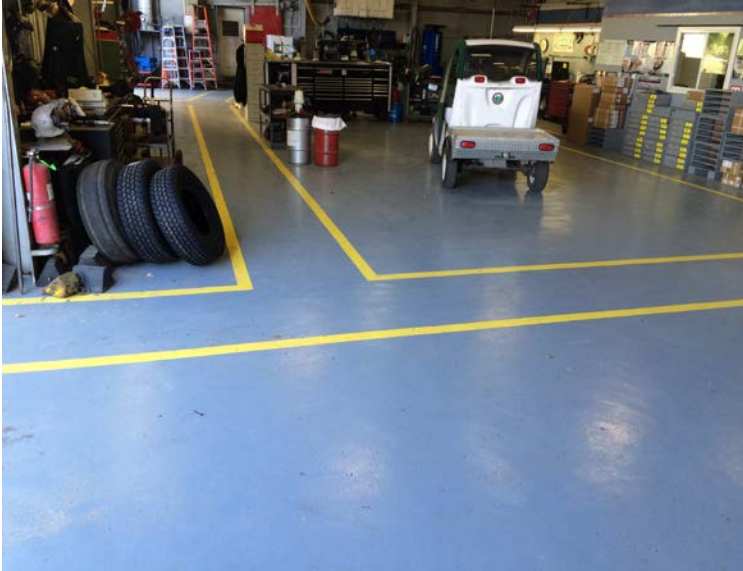
Line striping in safety yellow and floor back in service
