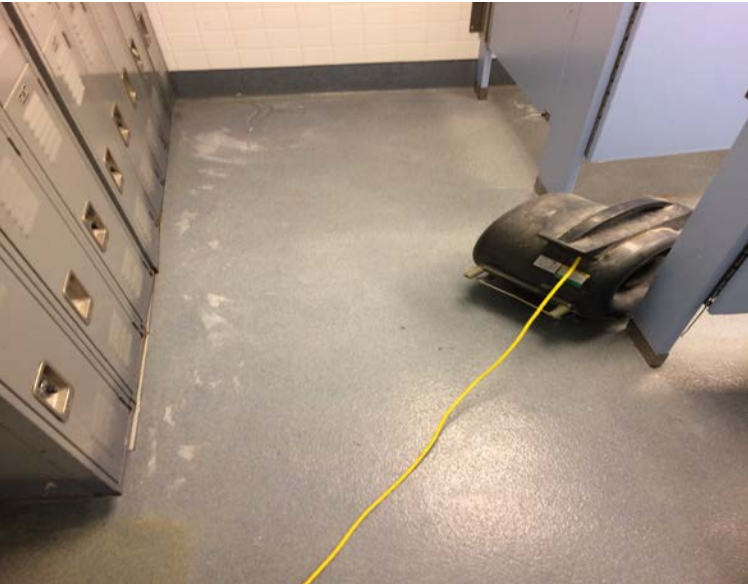
Thick coat of medium viscosity 100% solids epoxy, color Twilight Blue
