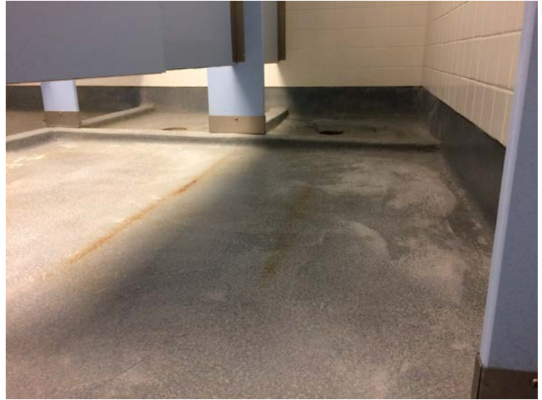
Wiped down with solvent & install masking tape on outer perimeter
