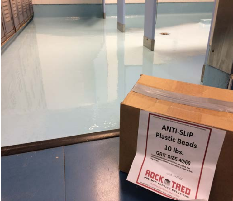
Integrate rubber beads for anti-slip while comfortable for bare feet.
