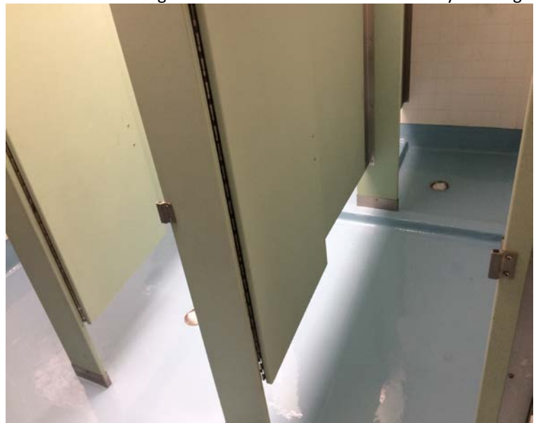
Anti-bacterial coating with much smoother surface for easy cleaning
