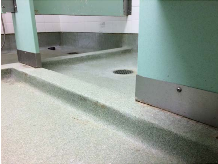
Dry blow substrate after thorough scrubbing with Rock-Solv cleaner
