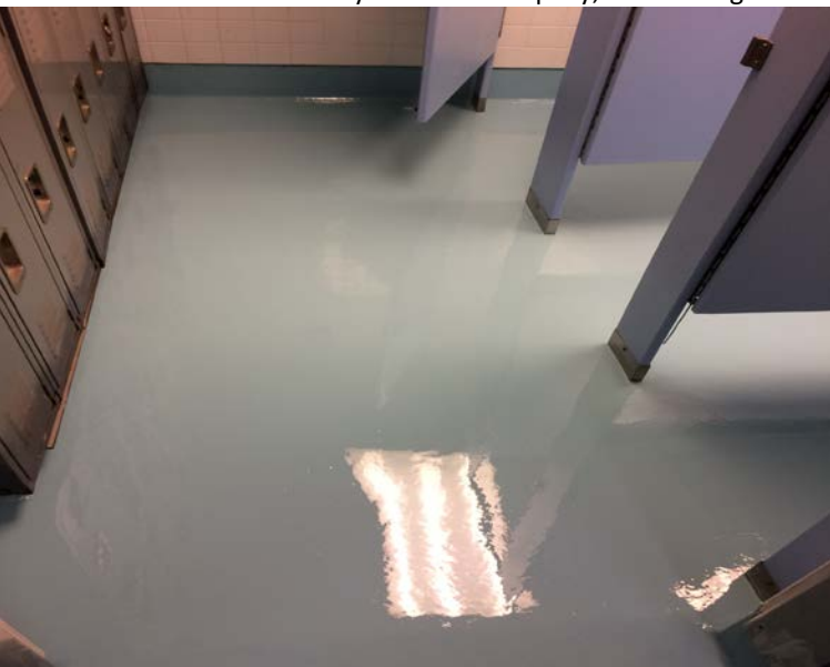
Thick coat of medium viscosity 100% solids epoxy, color Twilight Blue
