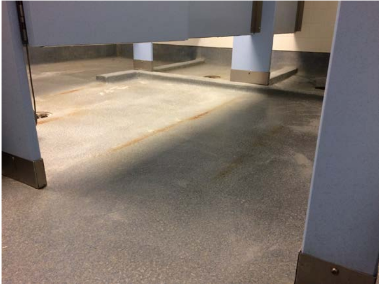
Integrate rubber beads for anti-slip while comfortable for bare feet.
