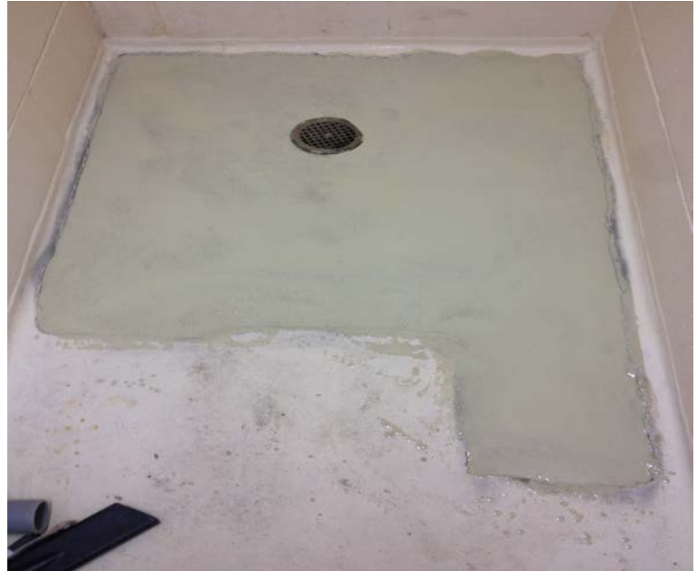
Recoat whole area to properly seal with off-white chemical resistant topcoat & medium non-skid texture
