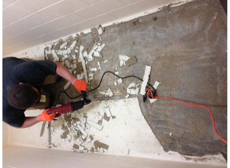
After repairs & drying substrate a 3-part cementitious urethane coat
