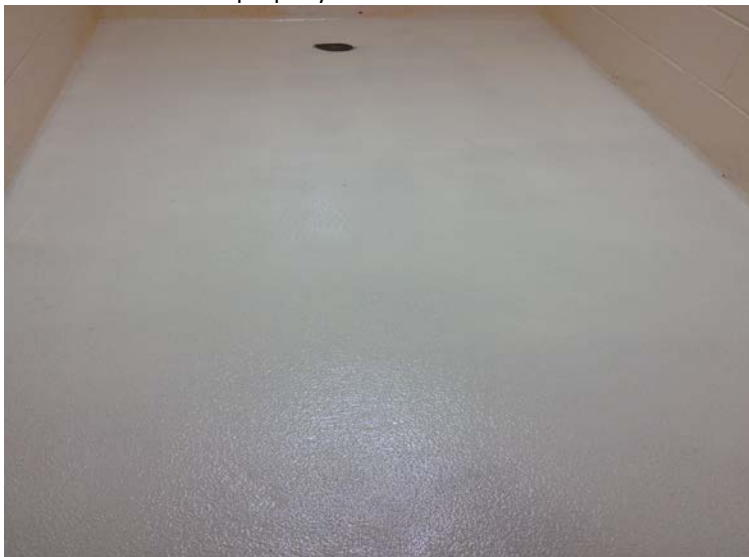
Recoat whole area to properly seal with off-white chemical resistant topcoat & medium non-skid texture
