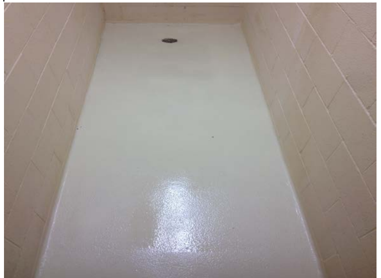
Recoat whole area to properly seal with off-white chemical resistant topcoat & medium non-skid texture
