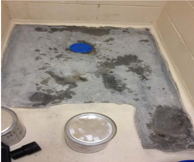
Recoat whole area to properly seal with off-white chemical resistant topcoat & medium non-skid texture
