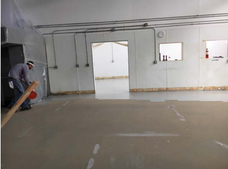
All cracks & imperfections filled & prepared prior to topcoat
