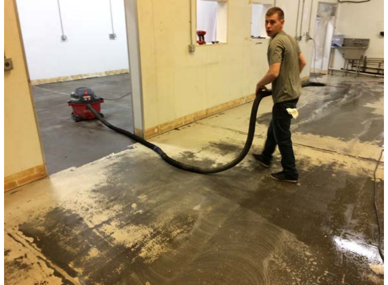
Lots of material removed & coarse profiling for superior bonding
