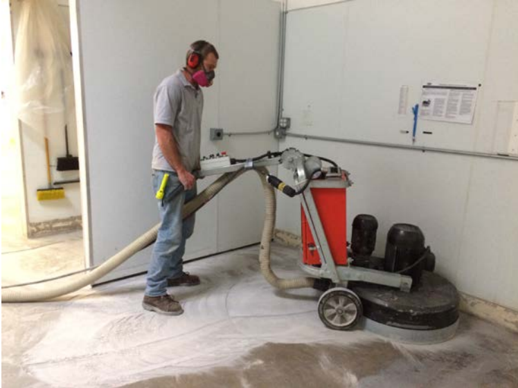
Detail grinding around drains & floor sinks
