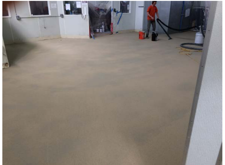
Base coat of cementitious urethane installed; remove excess sand
