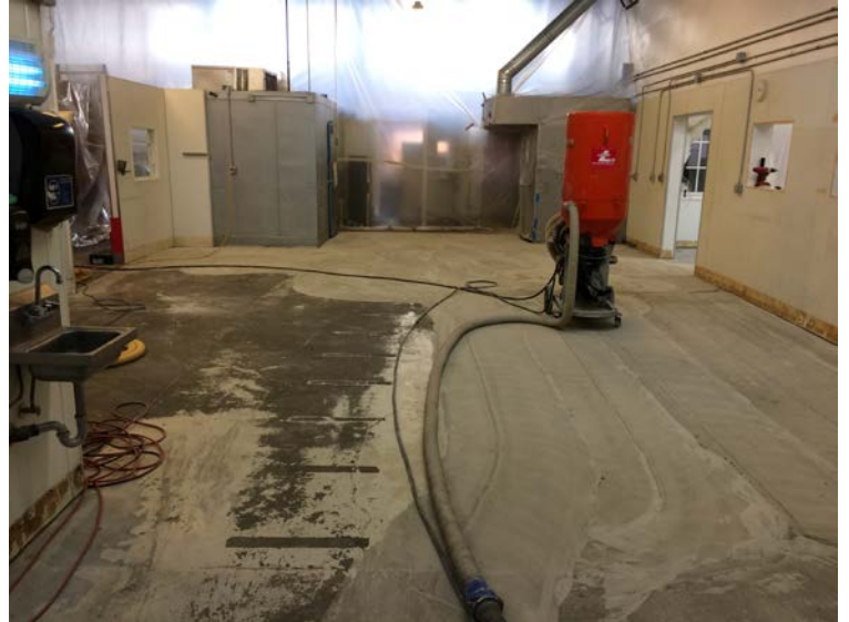
Base coat of cementitious urethane installed; remove excess sand
