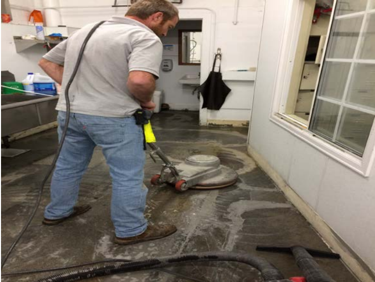
First pass of aggressive grinding with #30 grit diamonds
