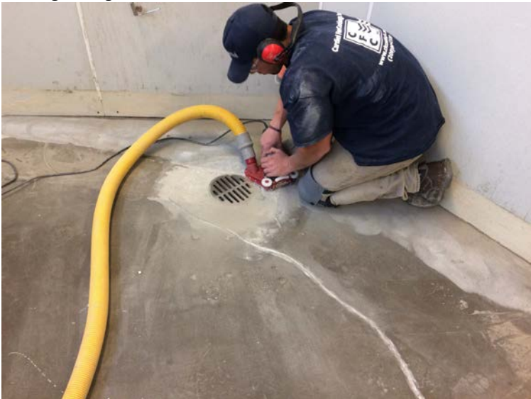
Detail grinding around drains & floor sinks
