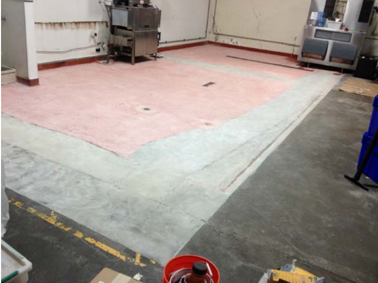
Three part cementitious urethane topcoat system for durability
