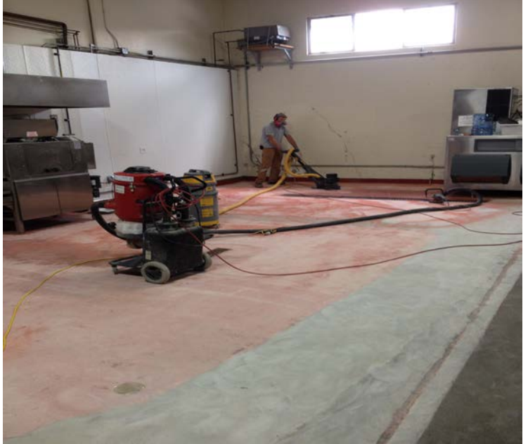
First application of cementitious urethane for superior bonding
