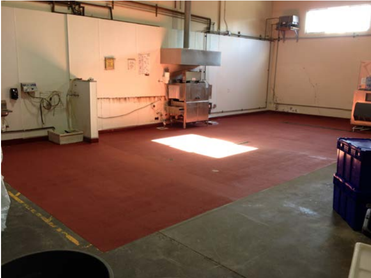
Three part cementitious urethane topcoat system for durability
