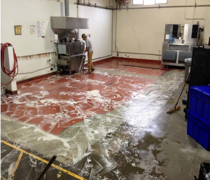
Area degreased, mechanically prepared & saw cut at ends
