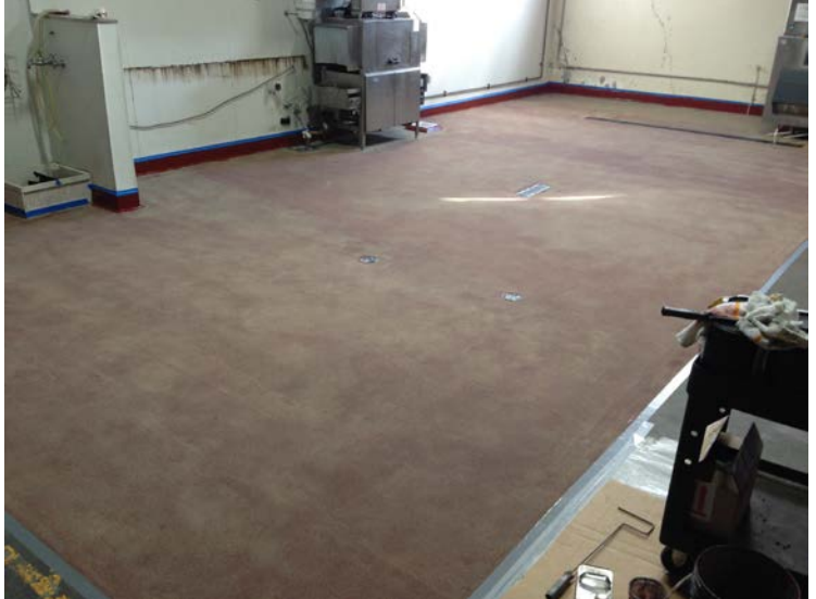
Aggressive non-skid profile makes this wash area slip resistant
