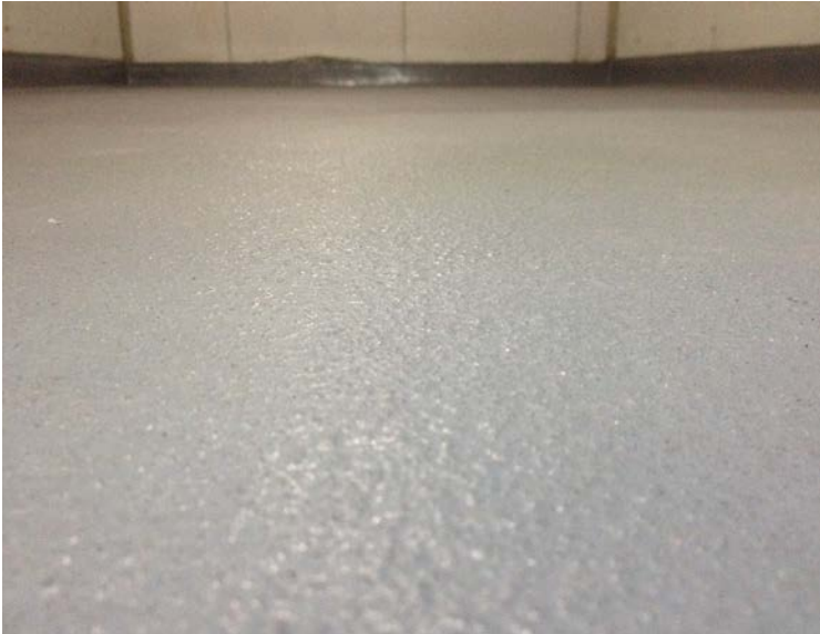
Medium non-skid texture with 30-grit aggregate medium
