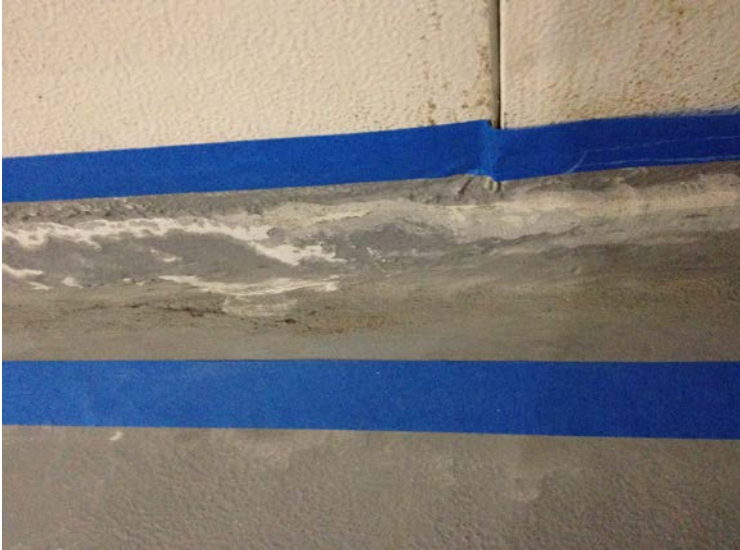
Medium non-skid texture with 30-grit aggregate medium
