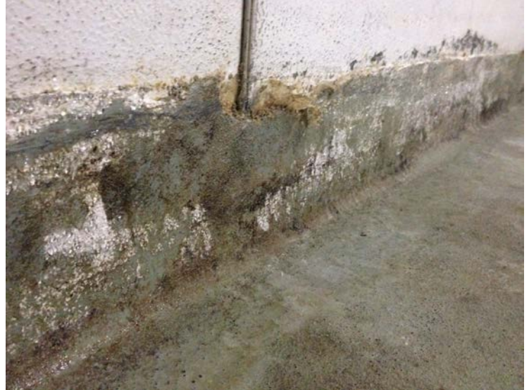
Cove base repaired & all recoated low viscosity epoxy
