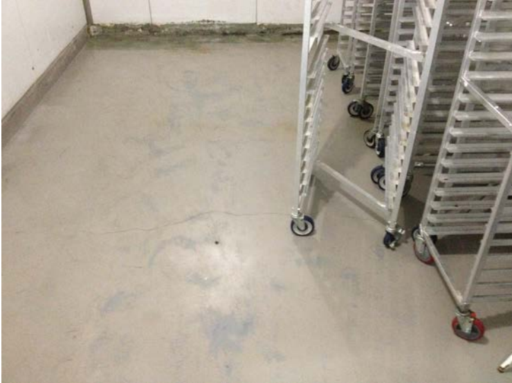
Cove base grinded down shows moisture from underneath
