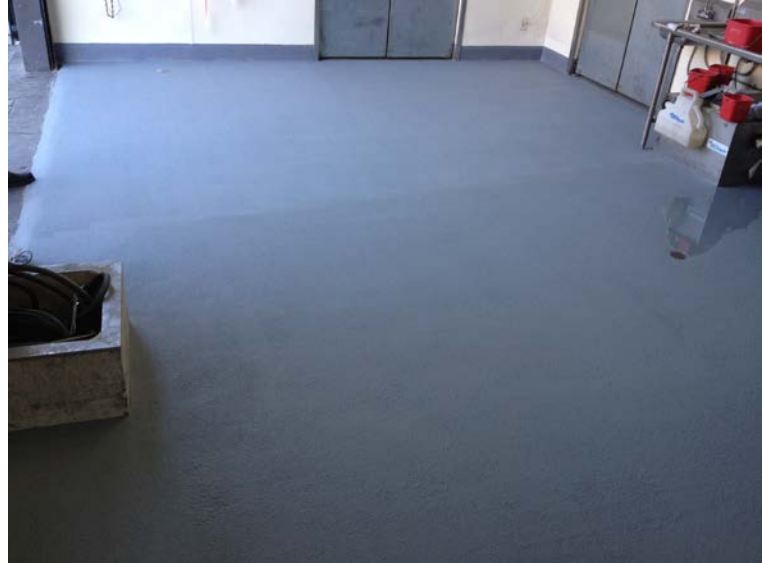
Two applications of urethane slurry mix will make this last
