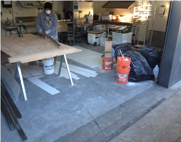
After dust barrier installation, diamond grind to clean substrate
