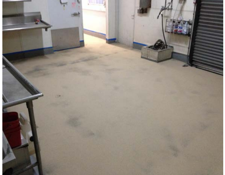
Two applications of urethane slurry mix will make this last
