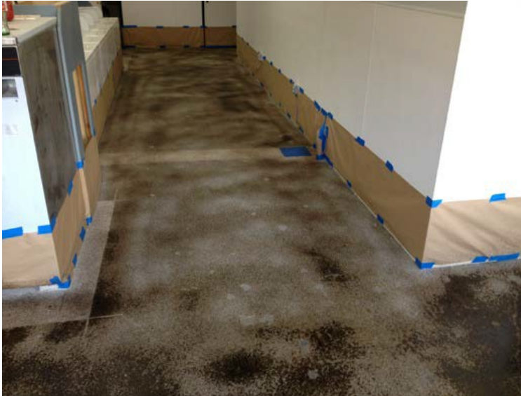
Multiple applications of Walnut stain penetrates deep in concrete.
