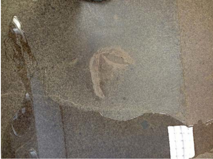
Multiple applications of Walnut stain penetrates deep in concrete.
