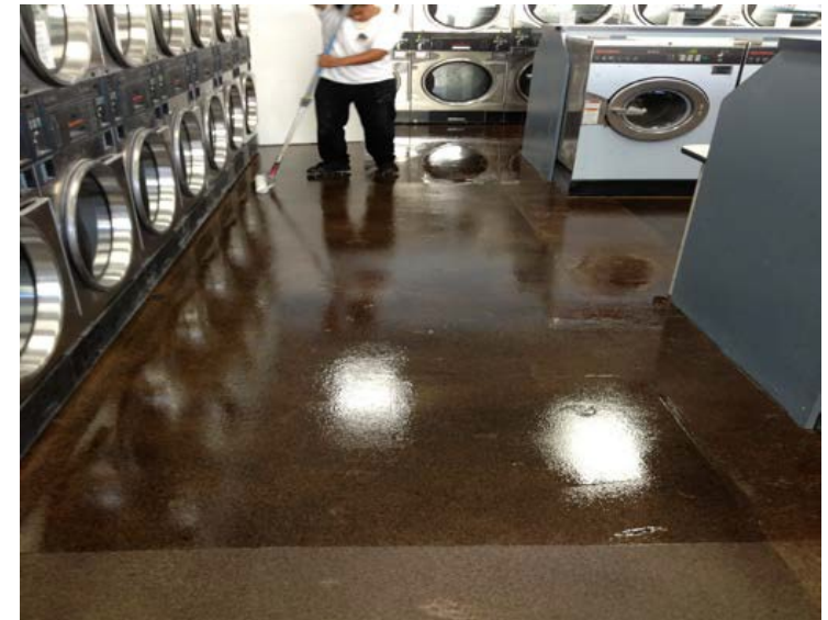
Finished with water-clear epoxy sealer and non-slip aggregate
