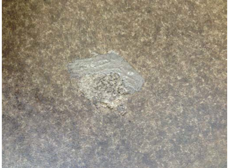
Finished with water-clear epoxy sealer and non-slip aggregate
