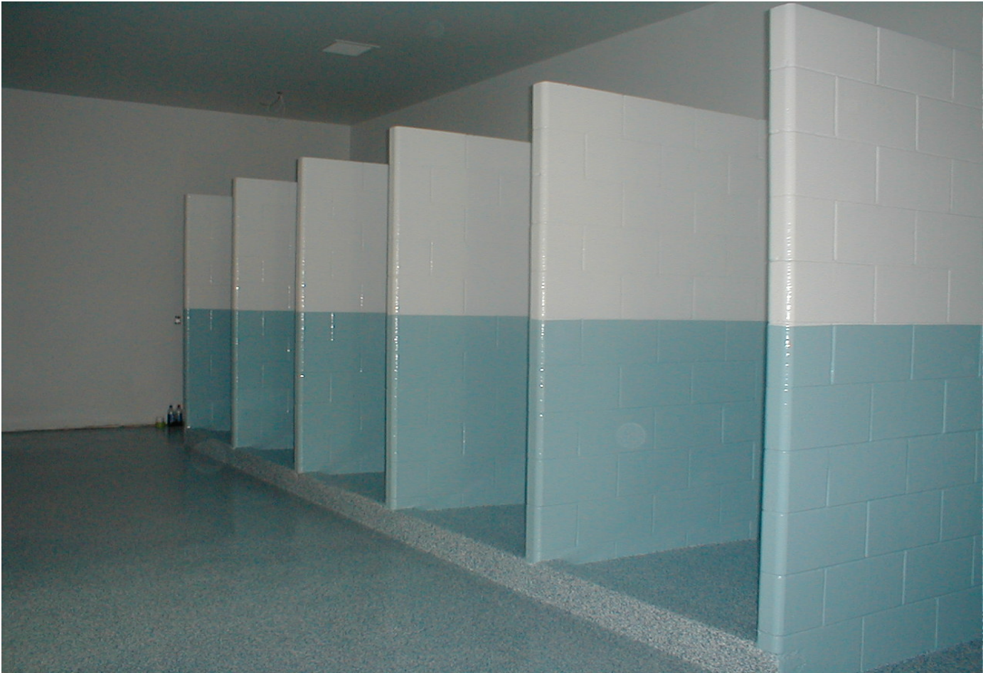
Chip system and wall coating for kennels, photo 2
