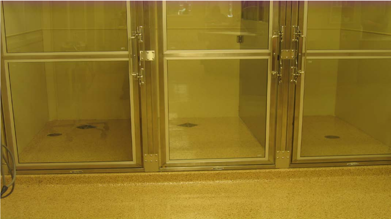
Chip system and wall coating for kennels, photo 1
