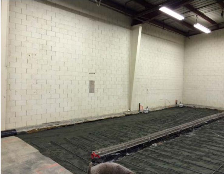
Ready for cement pour, ACO drains set in place
