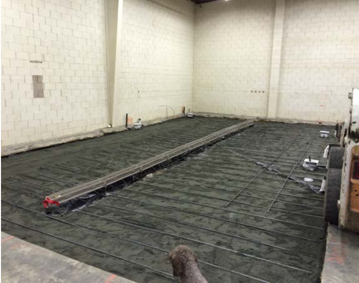
Ready for cement pour, ACO drains set in place
