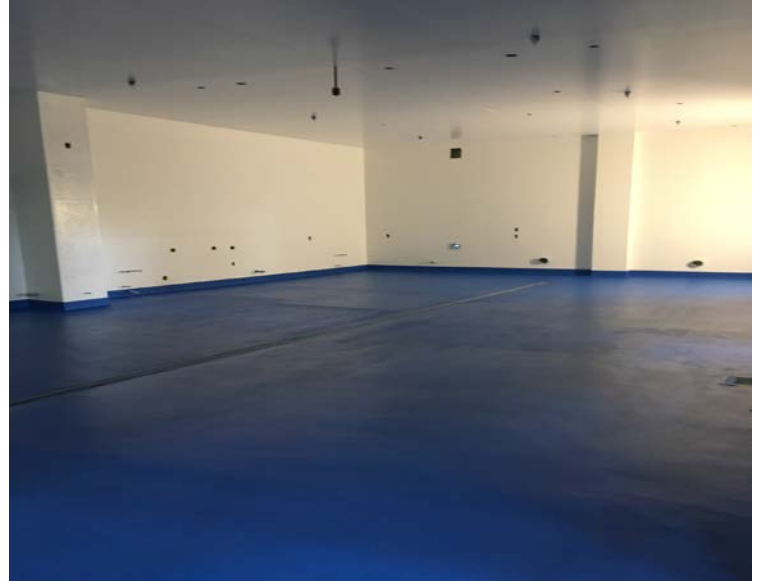
Walls w/epoxy & floors w/heavy duty cementitious urethane dressing
