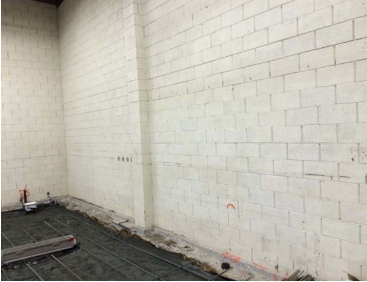
Cement block walls will be boxed in & finished with drywall
