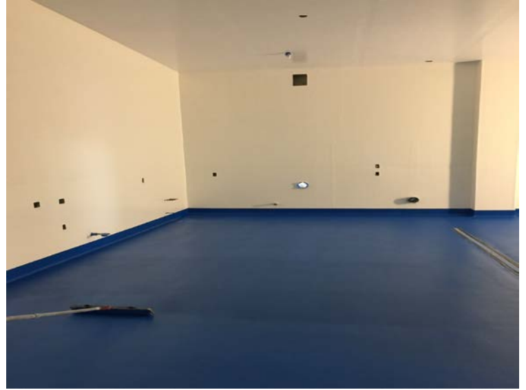
Floor consist of 1/4" trowel applied cementitious urethane slurry
