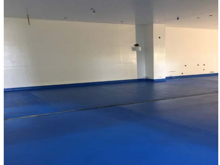
Walls w/epoxy & floors w/heavy duty cementitious urethane dressing
