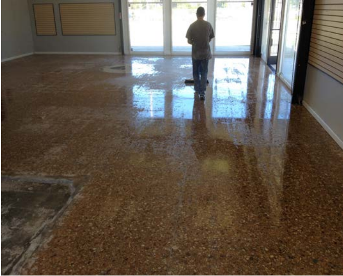
After 12 passes, 9 different grinding pads
