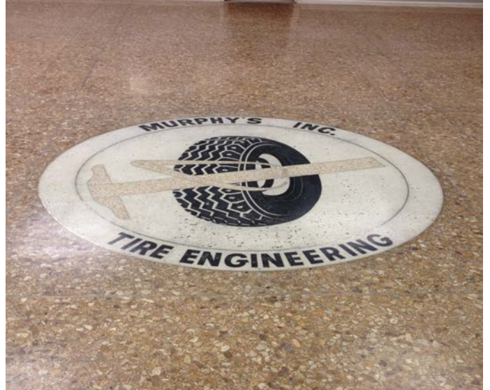
Completed with 1200 grit finish, all polished & easy to clean
