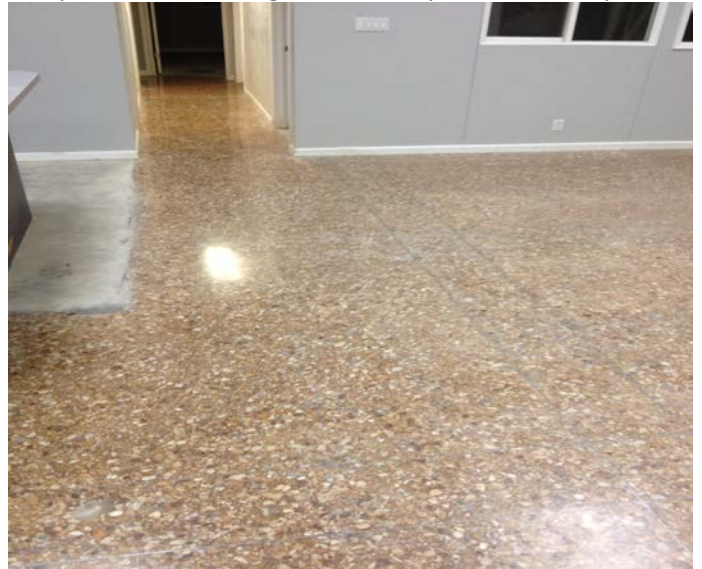
Completed with 1200 grit finish, all polished & easy to clean
