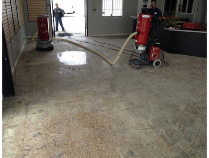
First passes with more aggressive 50-grit metal diamonds
