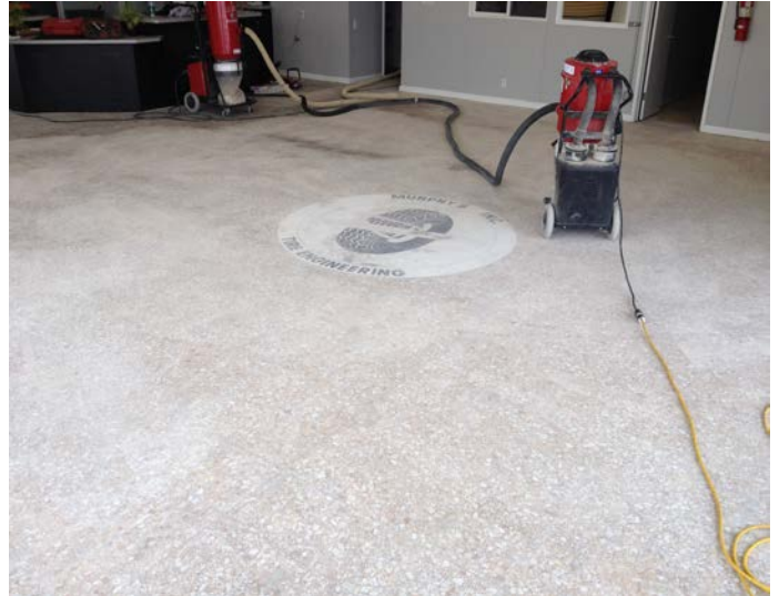
After 7 passes grinding & densifying, before final polish
