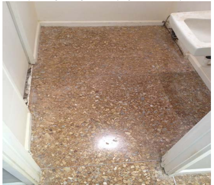
After 7 passes grinding & densifying, before final polish
