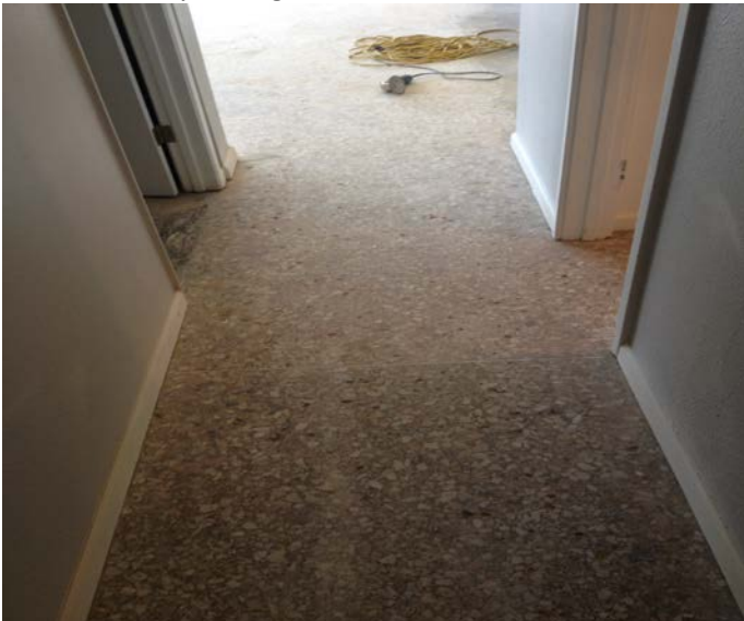
Restroom alley after glue removal
