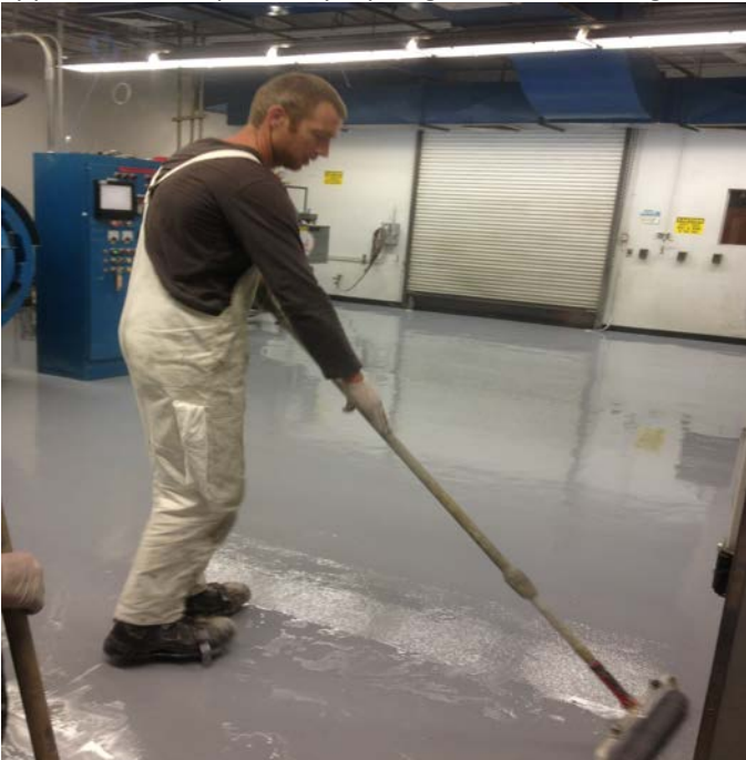
Application of top coat by squeegee & back-rolling
