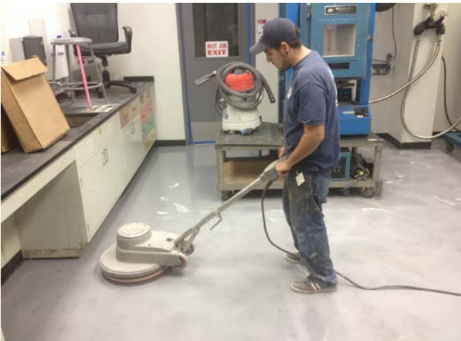
Sand screening with 80-grit after priming & more patching
