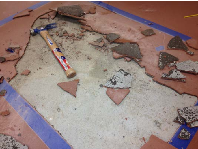
Repair area has been marked, edges diamond cut, failing system removed. Ready for surface preparation.
