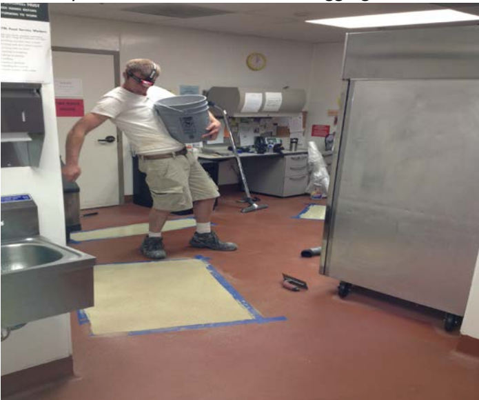
Urecon system installed with non-skid aggregate
