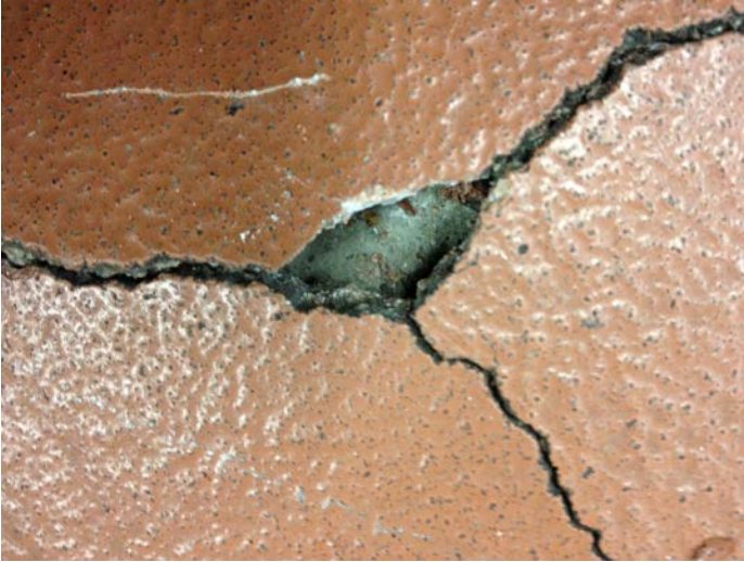
Repair area has been marked, edges diamond cut, failing system removed. Ready for surface preparation.
