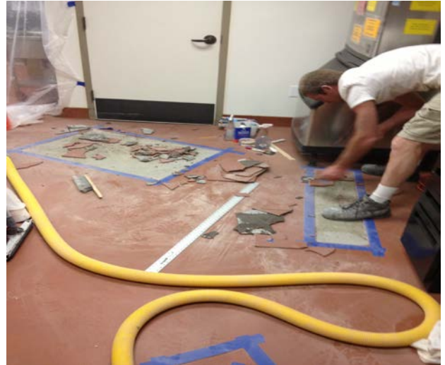
Repair area has been marked, edges diamond cut, failing system removed. Ready for surface preparation.
