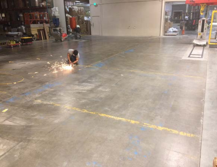
First slow pass with #30 grit diamonds for deep profiling
