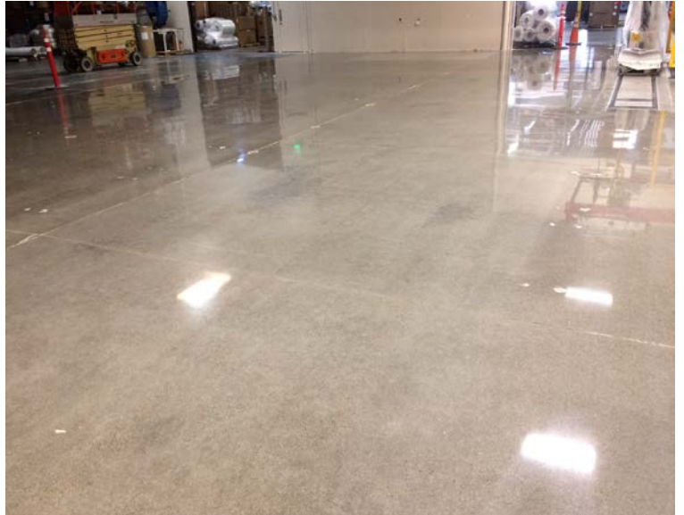
Nice aggregate exposure & high gloss after 8 steps of grinding & polishing, densifying, sealer application & high speed burnishing
