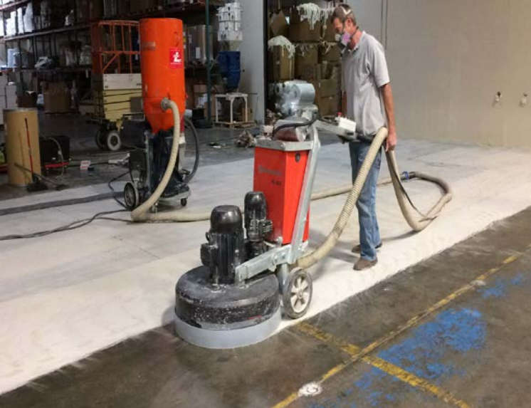
Nice aggregate exposure & high gloss after 8 steps of grinding & polishing, densifying, sealer application & high speed burnishing
