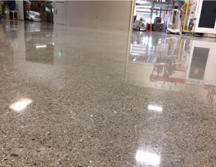
Nice aggregate exposure & high gloss after 8 steps of grinding & polishing, densifying, sealer application & high speed burnishing
