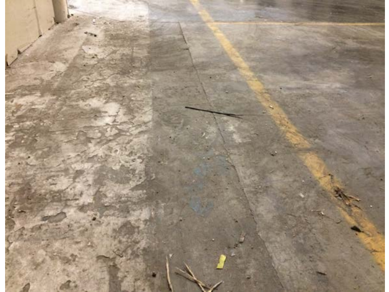
Open repair areas & remove contaminants for proper patch bonding
