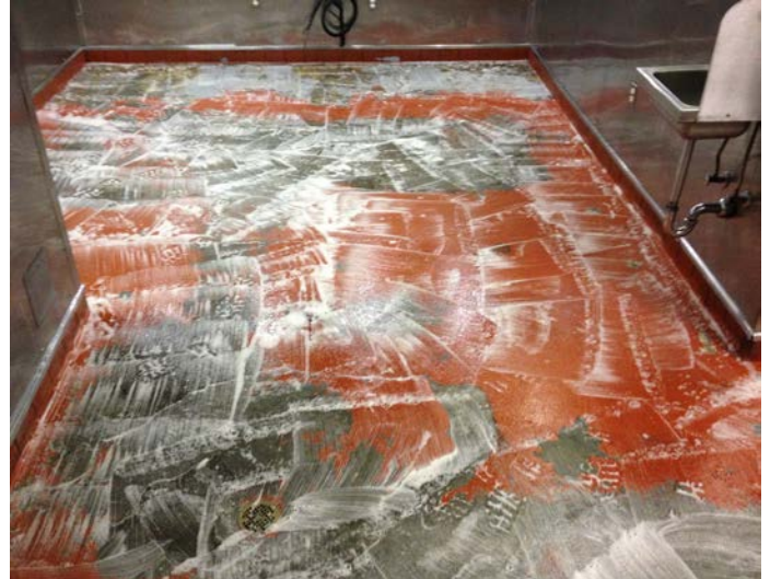
Multiple overlays applied & repairs made over the years
