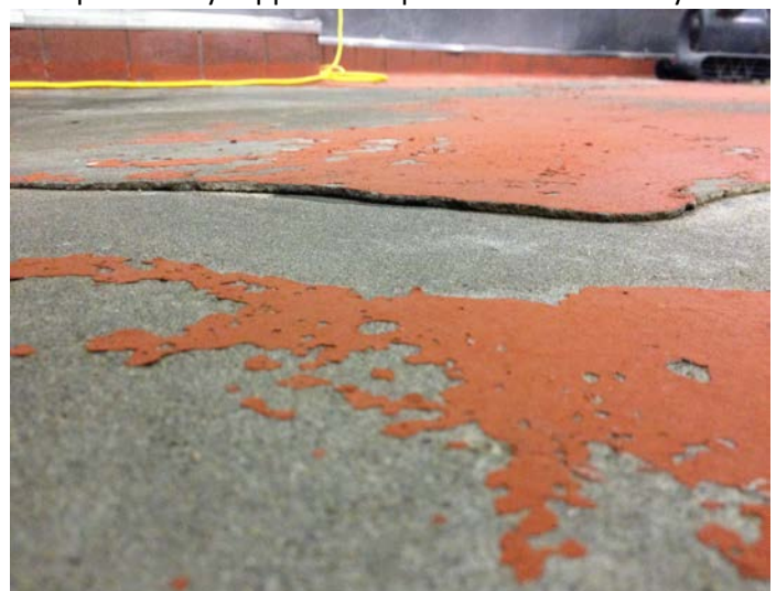
Multiple overlays applied & repairs made over the years
