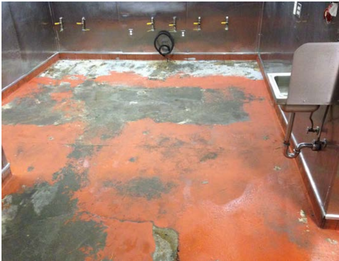
Substrate blow-drying after all contaminants removed
