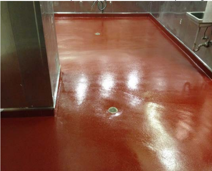
1/4" trowel down system, pigmented all the way through with slope to drains & 100% solids USDA/FDA compliant topcoat
