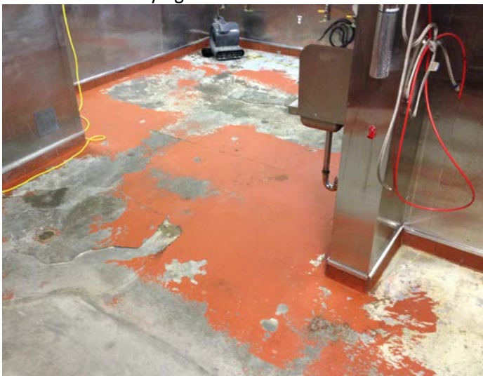
Substrate blow-drying after all contaminants removed
