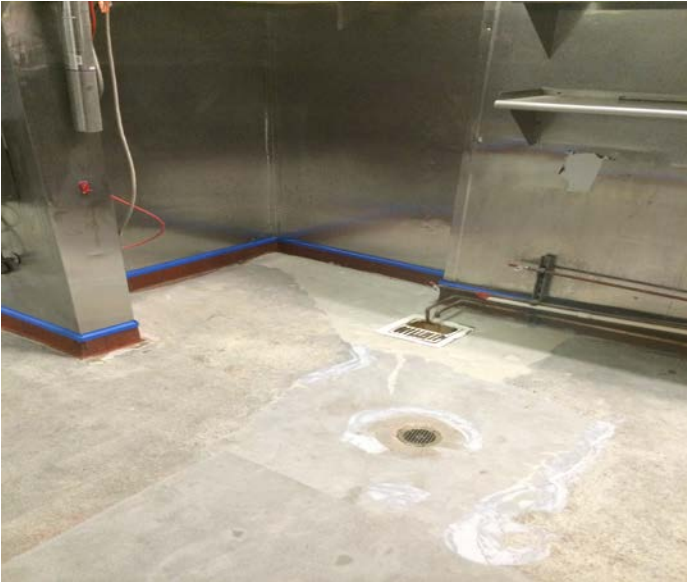
1/4" trowel down system, pigmented all the way through with slope to drains & 100% solids USDA/FDA compliant topcoat
