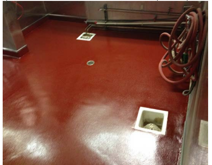
1/4" trowel down system, pigmented all the way through with slope to drains & 100% solids USDA/FDA compliant topcoat
