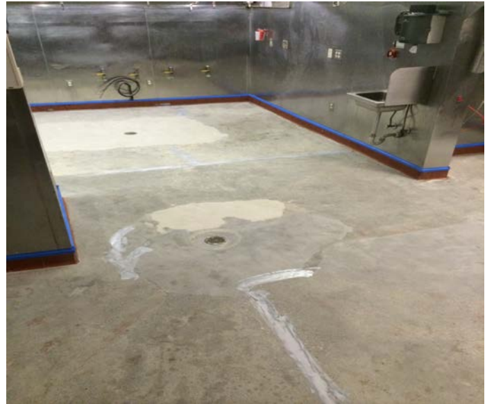
1/4" trowel down system, pigmented all the way through with slope to drains & 100% solids USDA/FDA compliant topcoat
