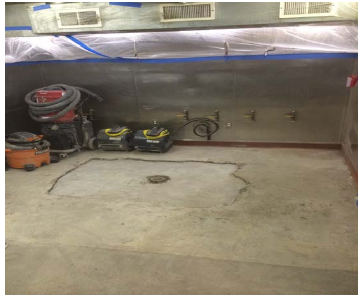
Seams and joints pre-filled as well, cove base primed
