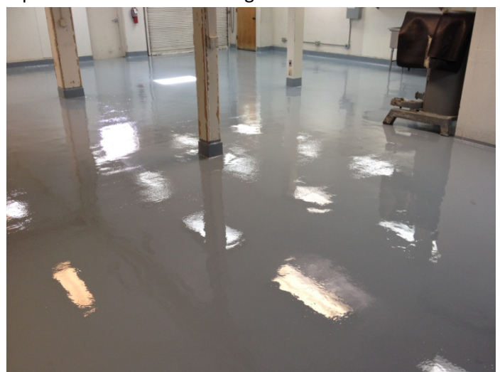
BASF Orange Peel textured topcoat for superior cleaning capabilities while maintaining non-skid characteristics
