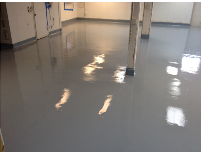
New cove base installed, primed, patched & top coated
