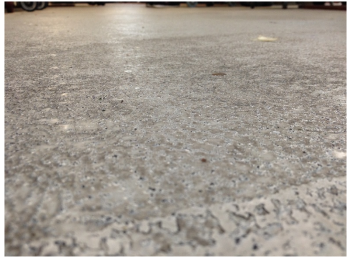
After cleaning, we sand screened area twice, ready for primer
