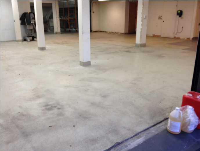
New cove base installed, primed, patched & top coated
