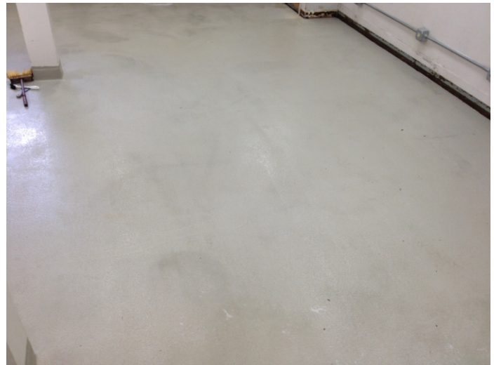
BASF Orange Peel textured topcoat for superior cleaning capabilities while maintaining non-skid characteristics
