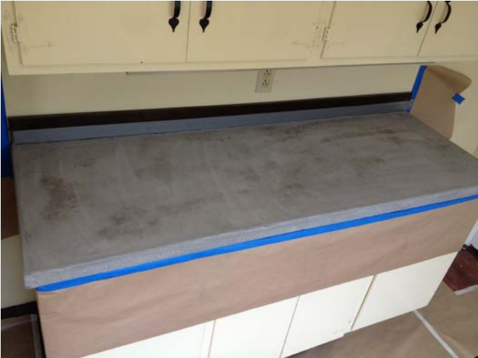
All sanded and prepped
