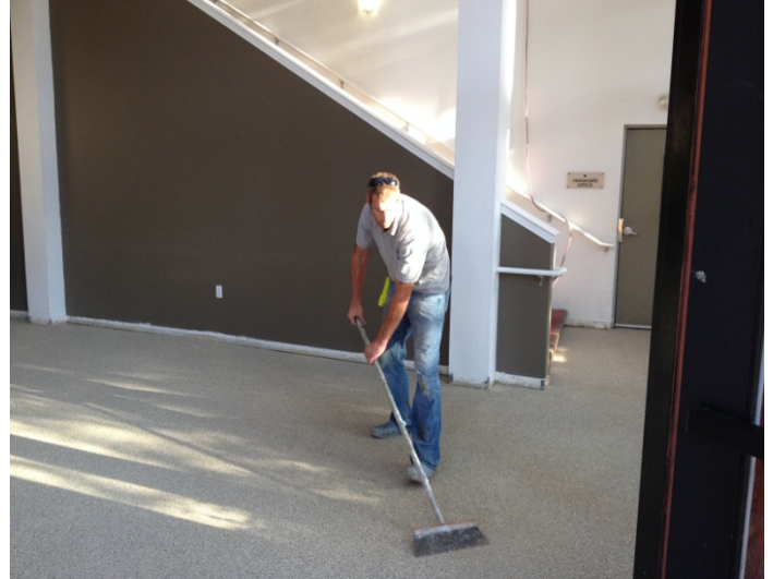
Water clear topcoat with full gloss when just installed
