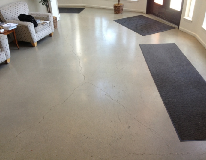
Whole area diamond grinded, cracks opened & patched
