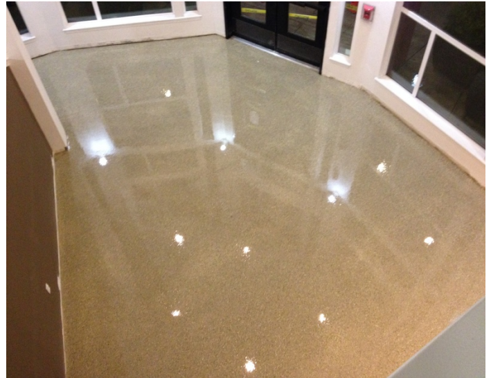
Water clear topcoat with full gloss when just installed
