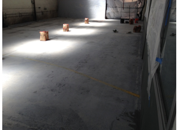
1/8" Cementitious urethane floor 'Gem Grey', medium non-skid Chemical, abrasion & impact resistant semi-gloss topcoat
