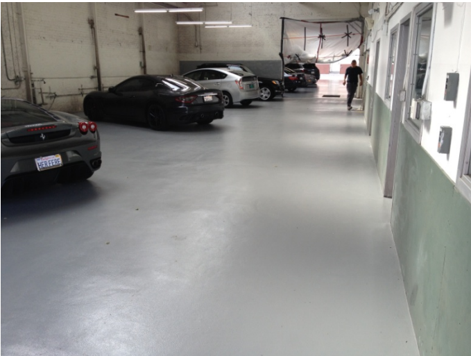
Moisture vapor tolerant system on floor, smooth on wall
