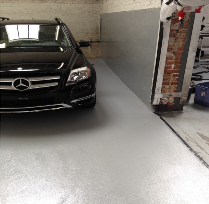
Moisture vapor tolerant system on floor, smooth on wall
